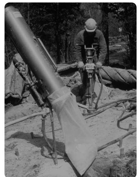
This image shows the first Dustcontrol solution of silica dust extraction in Sweden.
